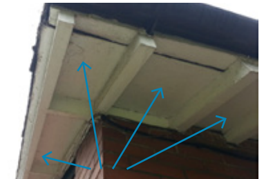
The soffit board is the horizontal board tucked away under the vertical fascia board, which is the long straight board that runs along the lower edge of the roof and often carries the guttering.
