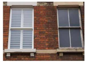
This imposing Victorian semi-detached villa required complete refurbishment, both inside and out. As well as brick-cleaning and repointing, stonework repair and new fascias, an important part of the project involved replacing the traditional box sash windows with modern, energy efficient, secure alternatives
