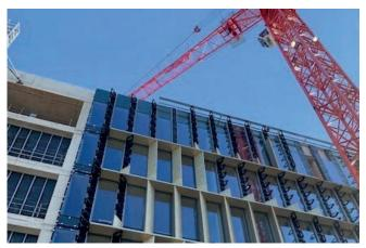
Perega was appointed to design the curtain walling and glass for this project. A feature of the façade was a frameless glass to glass joint to the Northwest corner, where two adjacent facades meet at an angle of 45 degrees.
