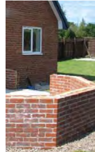
Dwarf wall built
