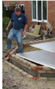
Insulation installed
