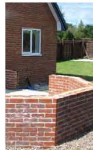
Dwarf wall built
