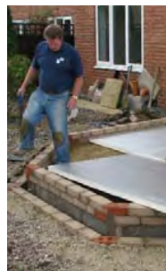
Insulation installed
